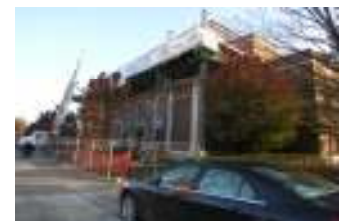
Pease exterior renovation work.
