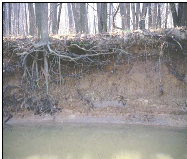
Undercut banks are a sign of flashy flows Photo: HRWC
